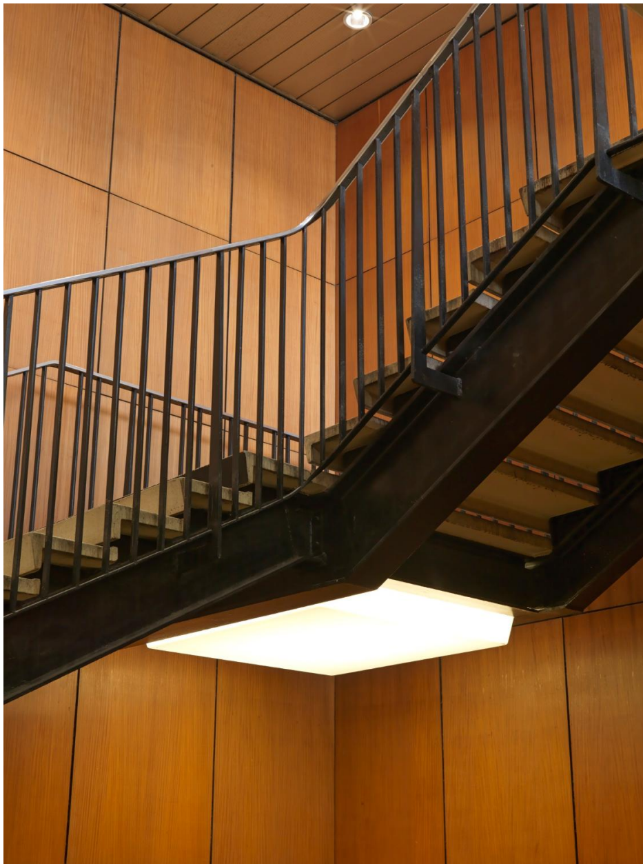
2018, circulation verticale: escalier ouest.
