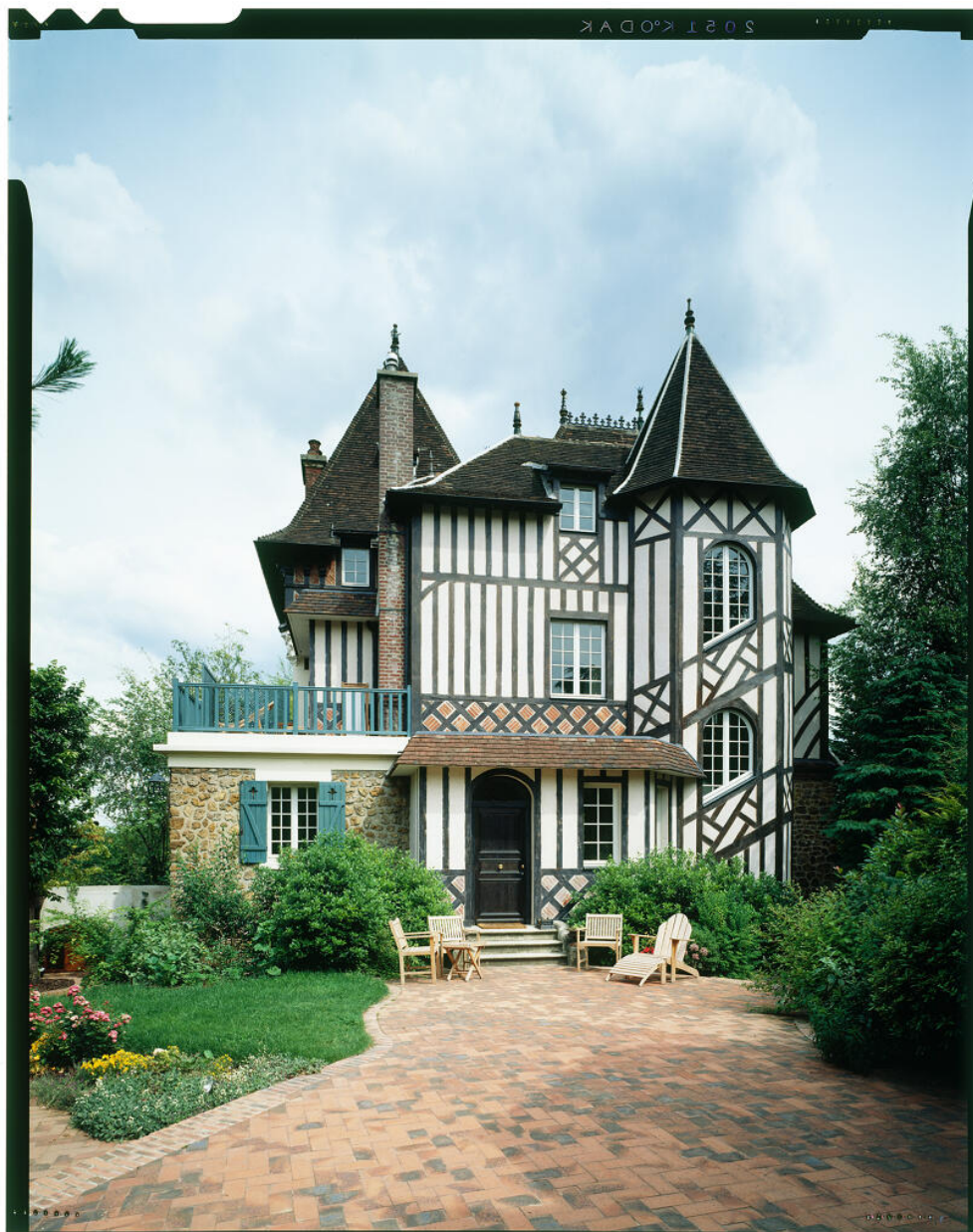
Villa dite "Mansion Clodoald", façade ouest
