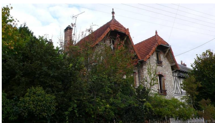
ETR252 (8, route de Chauffour)
