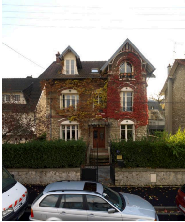
Façade principale. Phot. Philippe Ayrault IVR11_20167800697NUC4A
