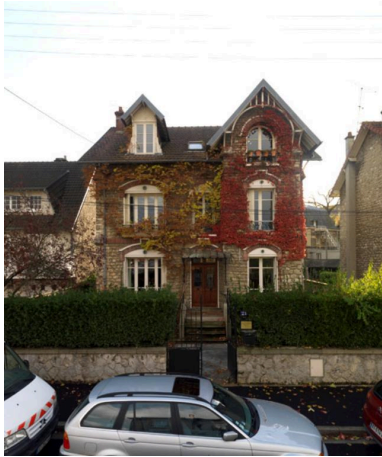
Façade principale. Phot. Philippe Ayrault IVR11_20167800697NUC4A
