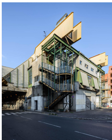
Patinoire de Saint-Ouen. Phot. Dupuid Augustin IVR11_20219300953NUC4A
