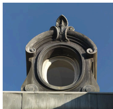
Lucarne ovale couronnant la travée centrale. Phot. Philippe Ayrault IVR11_20089100213NUC4A
