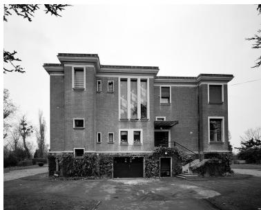
Façade Ouest. Phot. Vialles Jean-Bernard IVR11_19927800941V
