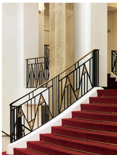
Hall-foyer Phot. Stéphane Asseline IVR11_20177500280NUC4A
