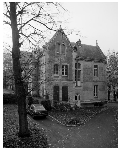
Façade nord Phot. Vialles Jean-Bernard IVR11_19919202695X
