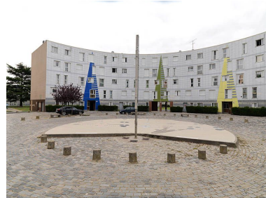
Place de l'Astrolabe. Phot. Stéphane Asseline IVR11_20129100057NUC4A
