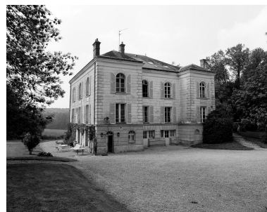
La façade est. Phot. Vialles Jean-Bernard IVR11_19917800284X
