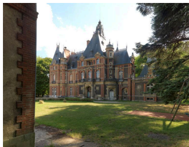
Façade principale. Phot. Laurent Kruszyk IVR11_20179500377NUC4A
