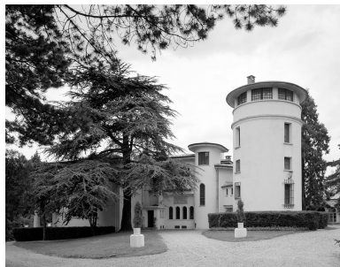
Façade principale (Est) Phot. Jean-Bernard Vialles IVR11_19919200786V
