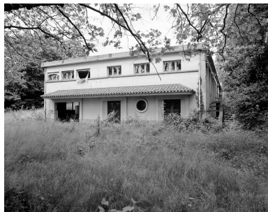
Façade sud du gymnase. Phot. Jean-Bernard Vialles IVR11_19919200800X
