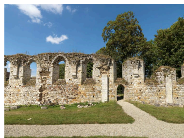
Mur gouttereau nord de la nef. Phot. Jean-Bernard Vialles IVR11_20167700163NUC4A
