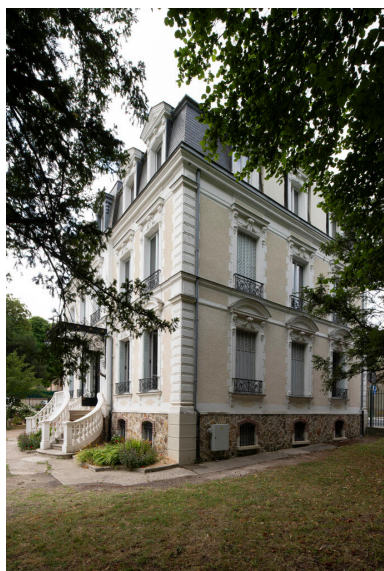
Angle nord. Repro. Ayrault Philippe, Phot. Ayrault Philippe IVR11_20239500657NUC4A
