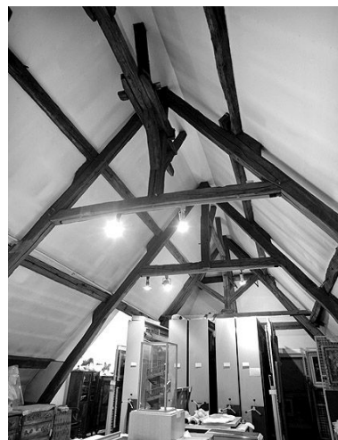
La charpente. Phot. Stéphane Asseline IVR11_20047700482X
