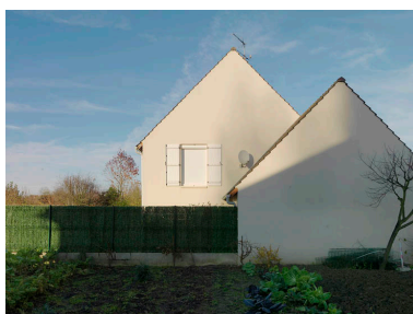
Survilliers. Zone pavillonnaire. Phot. Philippe Ayrault IVR11_20149500055NUC4A
