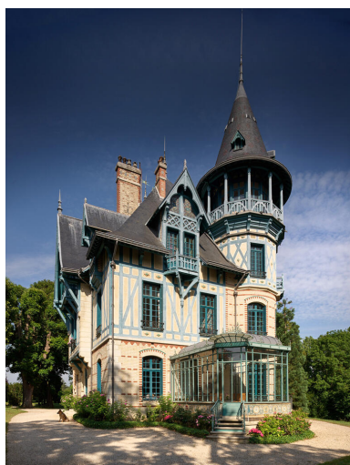
Vue générale, façade est. Phot. Asseline Stéphane IVR11_20207800333NUC4A
