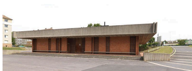
Façade ouest. Phot. Stéphane Asseline IVR11_20097701085NUC4A
