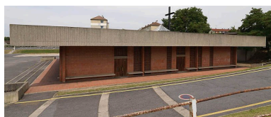
Façade sud. Phot. Stéphane Asseline IVR11_20097701087NUC4A
