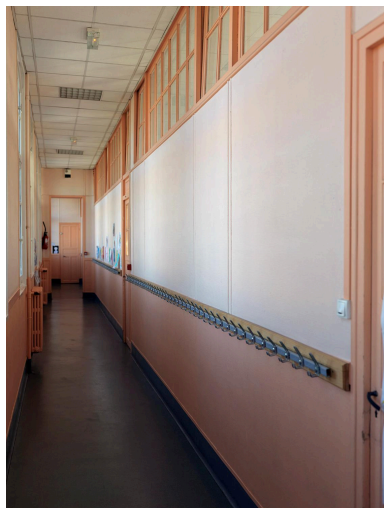
Couloir desservant les classes. Phot. Jean-Bernard Vialles IVR11_20089300359NUC4A
