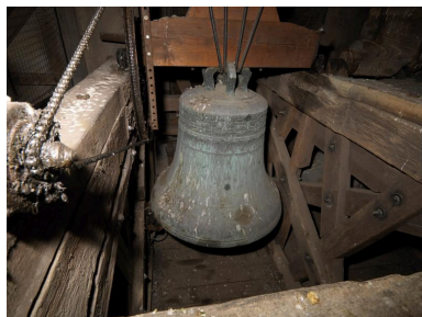
La cloche "Alexandrine" (1878). Phot. Jean-Bernard Vialles IVR11_20179500055NUC4A
