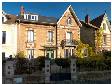
Façade principale. Phot. Laurent Kruszyk IVR11_20167800753NUC4A
