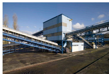
Parc a charbon. Manutention. Phot. Philippe Ayrault IVR11_20087700469NUC4A
