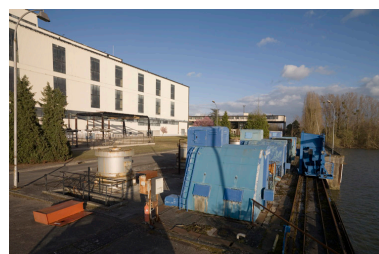
Stations de pompage. Phot. Philippe Ayrault IVR11_20087700454NUC4A
