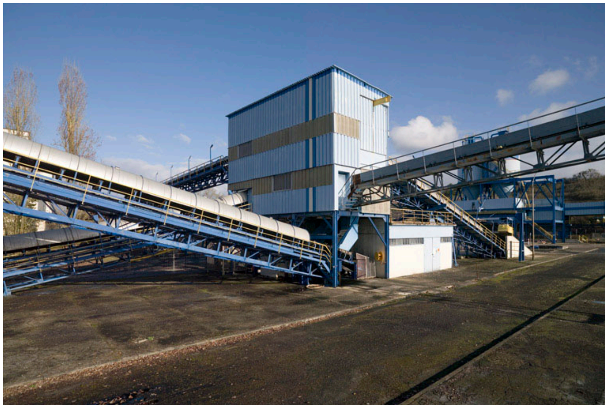
Parc a charbon. Manutention.
