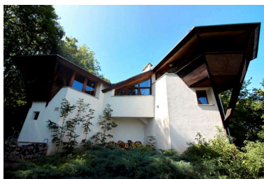
Facade postérieure. Phot. Eric Jacquard IVR11_20177300018NUC4A
