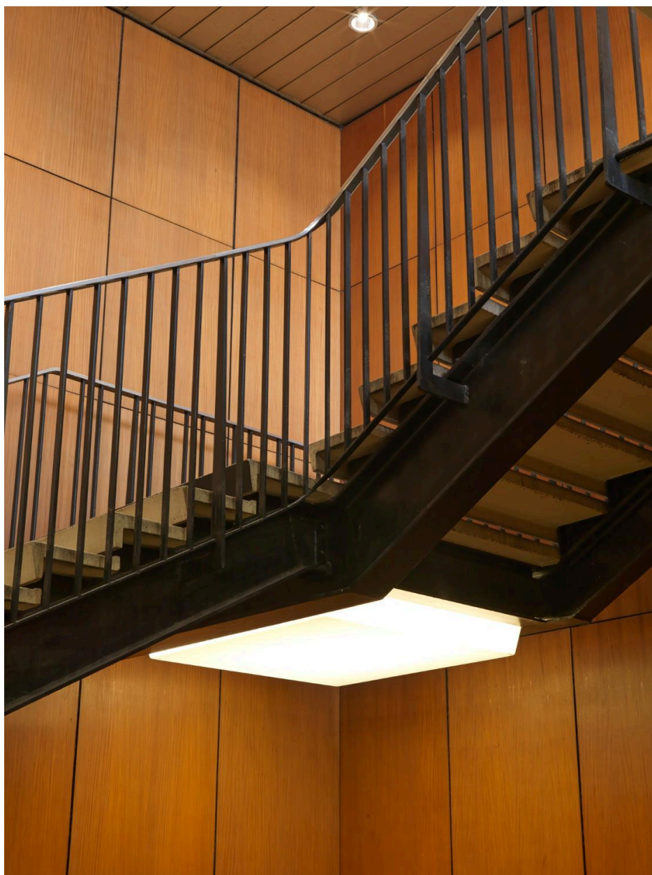
2018, circulation verticale: escalier ouest.
