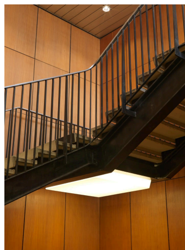
2018, circulation verticale: escalier ouest. Phot. Stéphane Asseline IVR11_20209400206NUC4A
