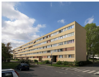
La barre M. Phot. Jean-Bernard Vialles IVR11_20109100062NUC4A
