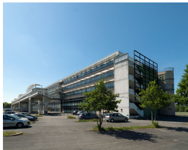
Vue est. Phot. Jean-Bernard Vialles IVR11_20157700053NUC4A
