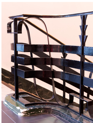
Main-courante, garde-corps, fer forgé, Raymond Subes Phot. Stéphane Asseline IVR11_20189200081NUC4A
