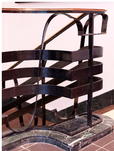
Main-courante, garde-corps, fer forgé, Raymond Subes Phot. Stéphane Asseline IVR11_20189200080NUC4A
